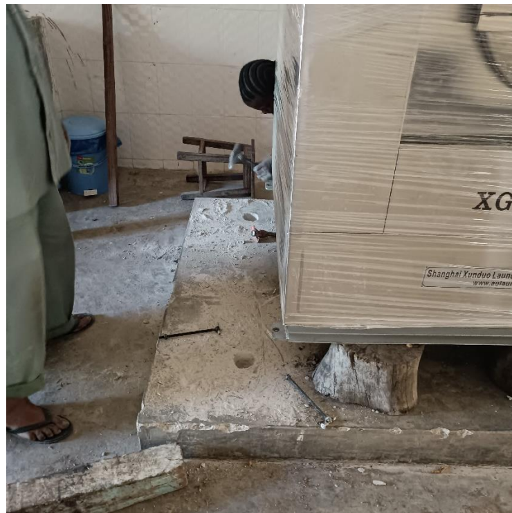
Fig 6: The process of making holes on the base to put bolt for tightening the machine.
