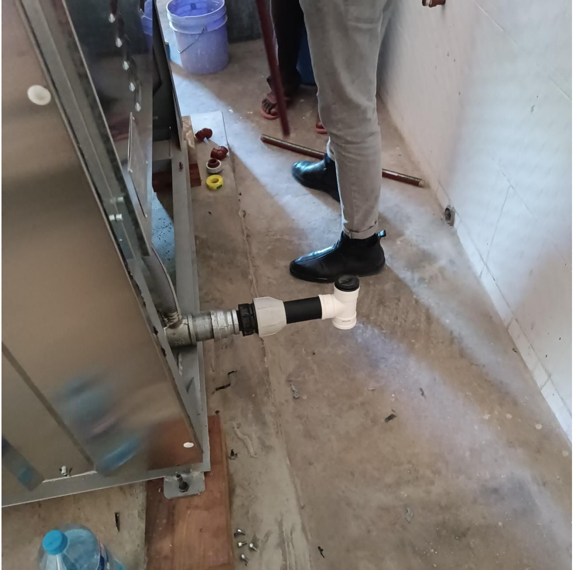
Fig 9: The process of installing water system to the machine
