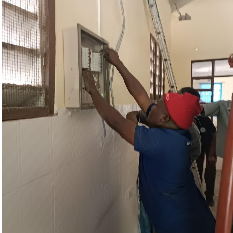
Fig 11: The process of installation of 3 phase main switch with socket breaker
