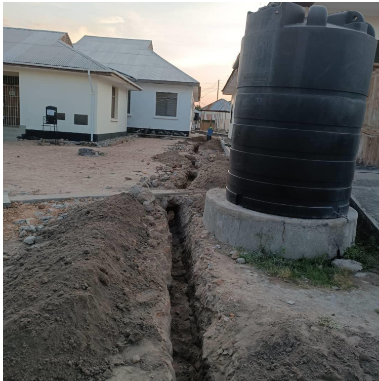
Fig 5: Trenches for laying pipes to CTC and Laboratory buildings
