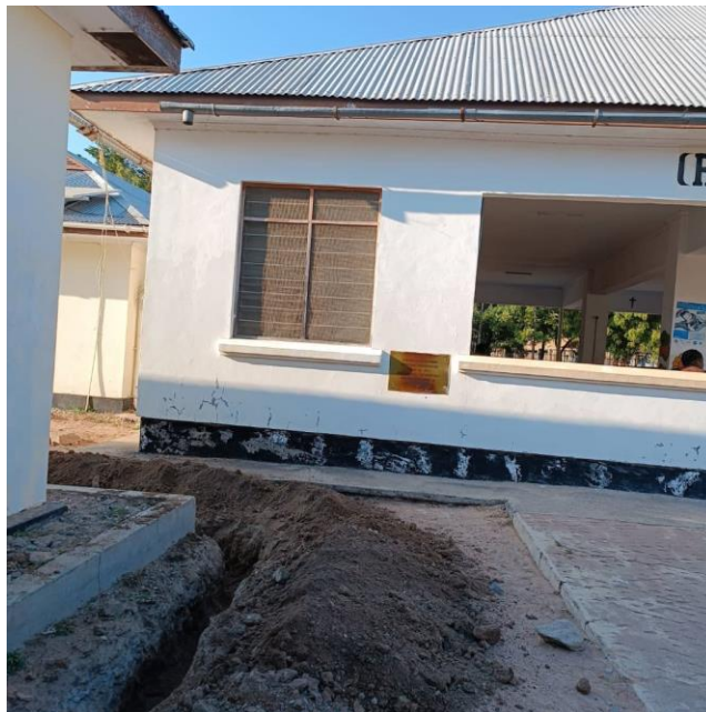
Fig 7: Trenches for laying pipes to RCH building
