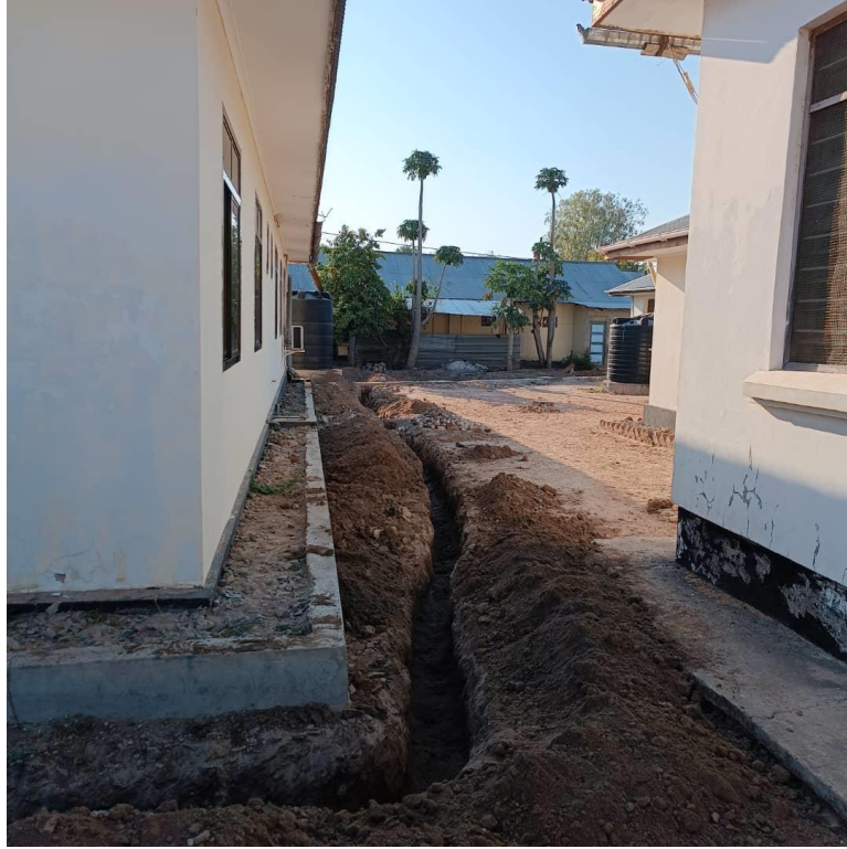
Fig 4: Trenches for laying pipes to laboratory buildings
