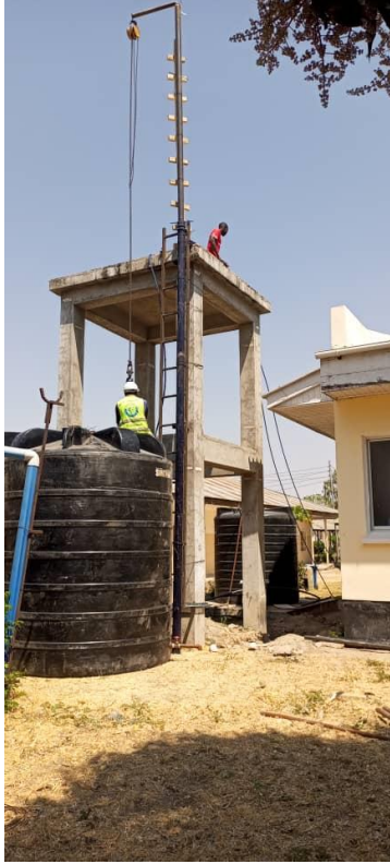
Fig 11: process of taking the 10,000 litres tank to a tower.
