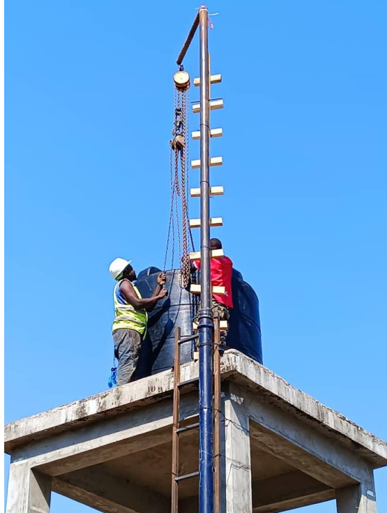
Fig 13: process of taking the 10,000 litres tank to a tower
