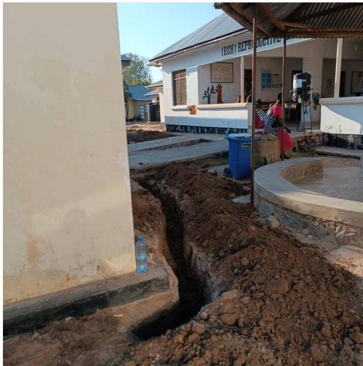
Fig 3: Trenches for laying pipes to OPD buildings.
